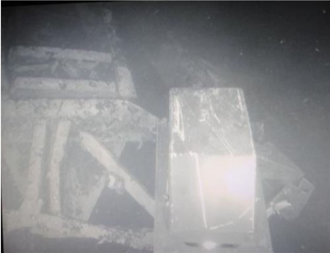
Shear in action cutting through deck beams
